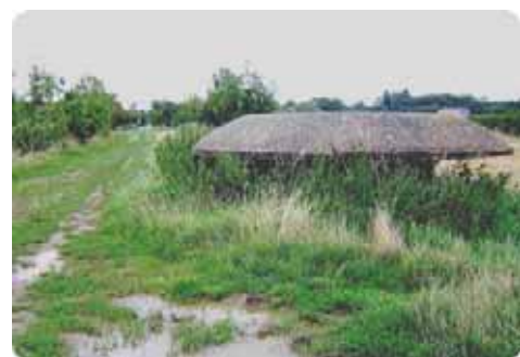
A cantilevered 'Oakington' type pillbox. Photo courtesy of Peter Duthie, Rights of Way
