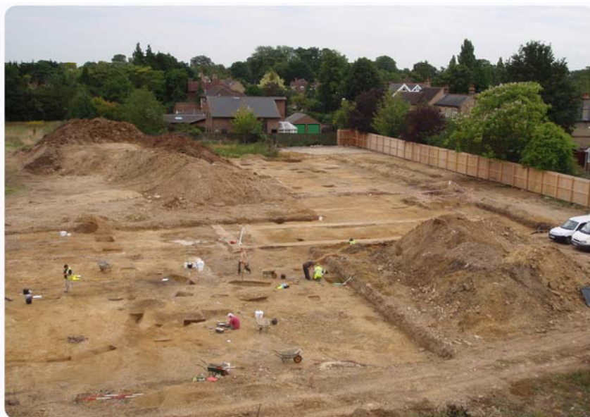
Excavations of the Iron Age roundhouse at Impington Lane, Impington (photo courtesy of Oxford Archaeology East).
