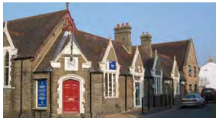
Change of use - the Town Council offices converted into a larger library in Littleport
