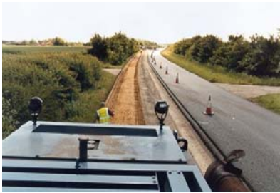
Carriageway reconstruction work
