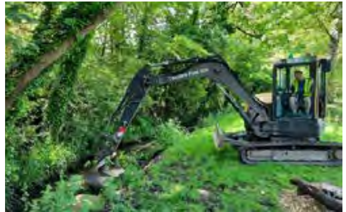
Re-shaping works on Vicar's Brook (Mungovan, 2021) Wild Trout Trust © R Mungovan
