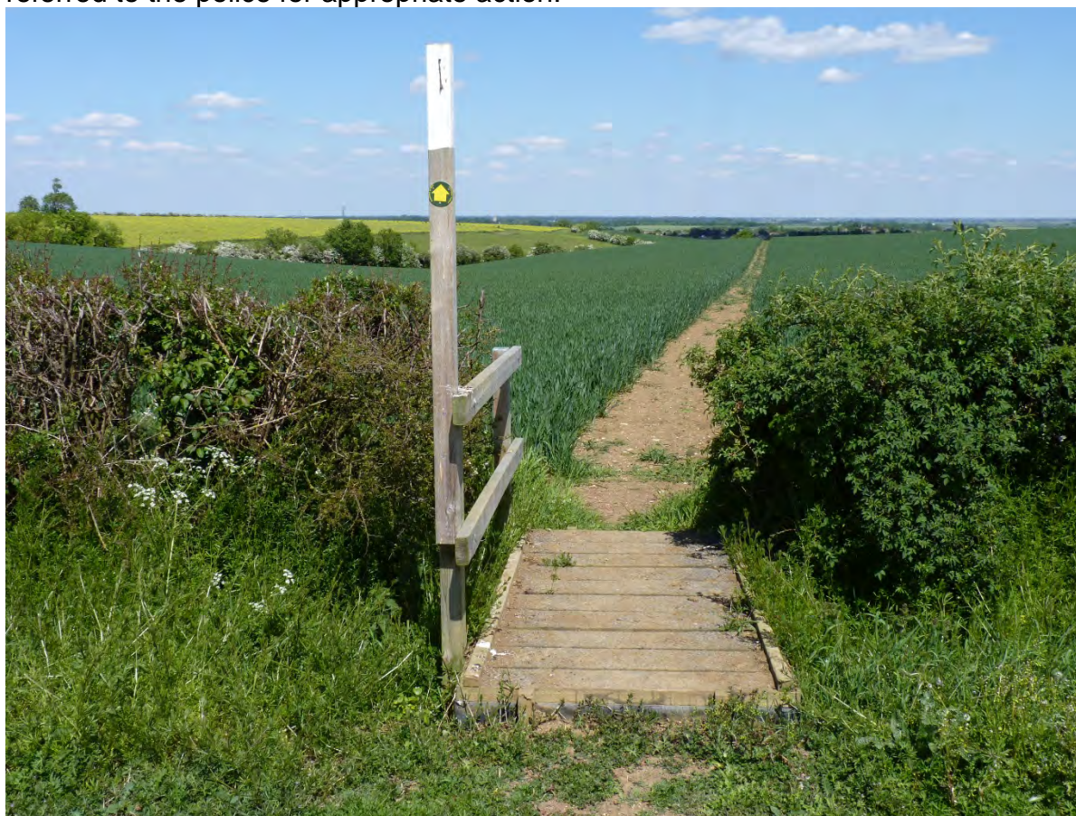
Bridge reinstatement Sawtry (Footpath 27)
