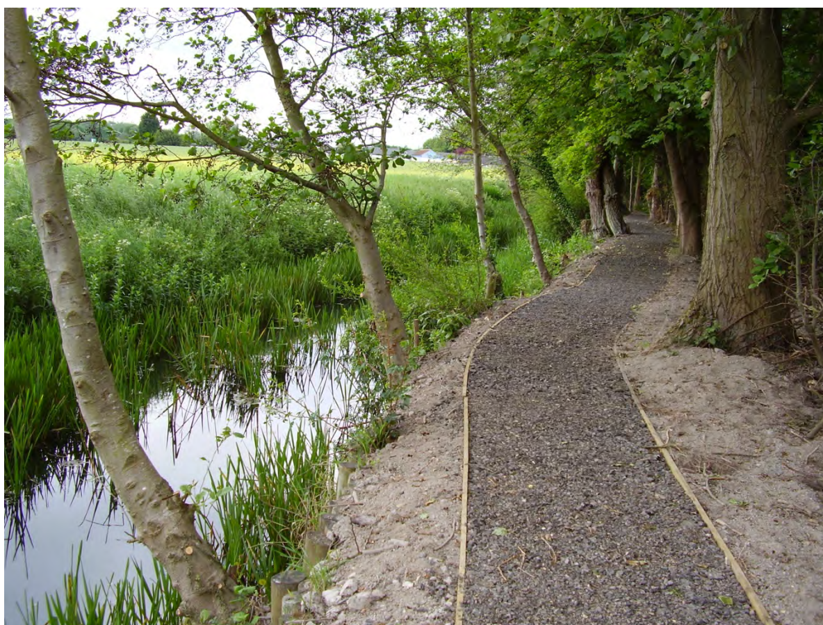
Shepreth footpath improvements
