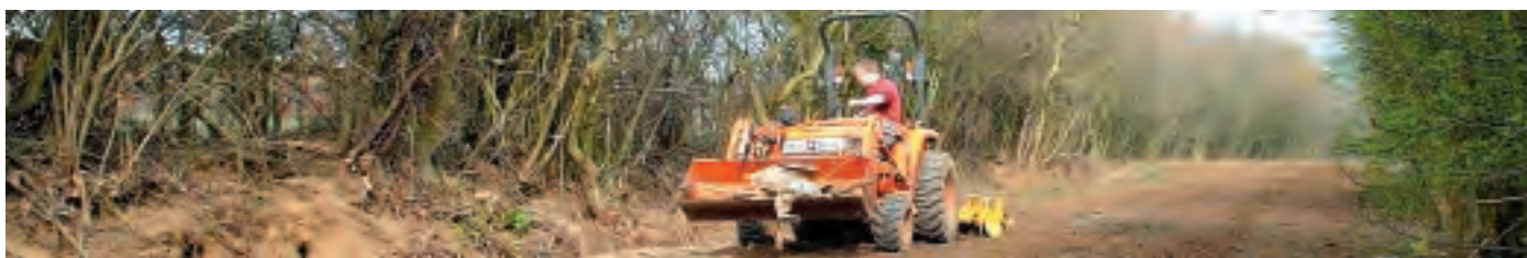
Byway improvements at Gypsy Lane Dullingham
