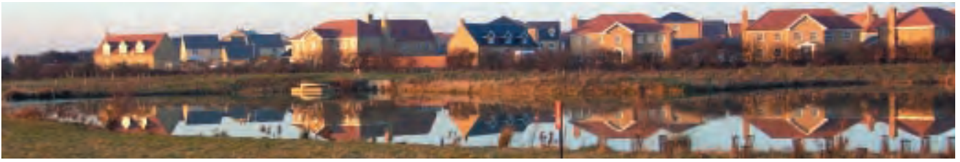
New housing at Cambourne by Caxton Bridleway 5
