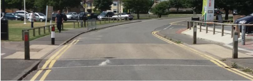
Speed tables are a raised section of road, with a ramp on both sides. The ramps are painted with white arrows to make them more obvious to motor vehicle drivers. The aim of the speed table is to slow motor vehicle traffic to a safe speed, as the ramps become uncomfortable for vehicle drivers if they are driven over too fast. A speed table is normally around 75mm high, and can vary in length.
