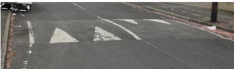
Speed humps have a short rounded top which is typically 75mm high. The ramps either side are painted with white arrows to make them more obvious to motor vehicle drivers. The aim of the speed hump is to slow motor vehicle traffic to a safe speed, as the ramps become uncomfortable for vehicle drivers if they are driven over too fast.
